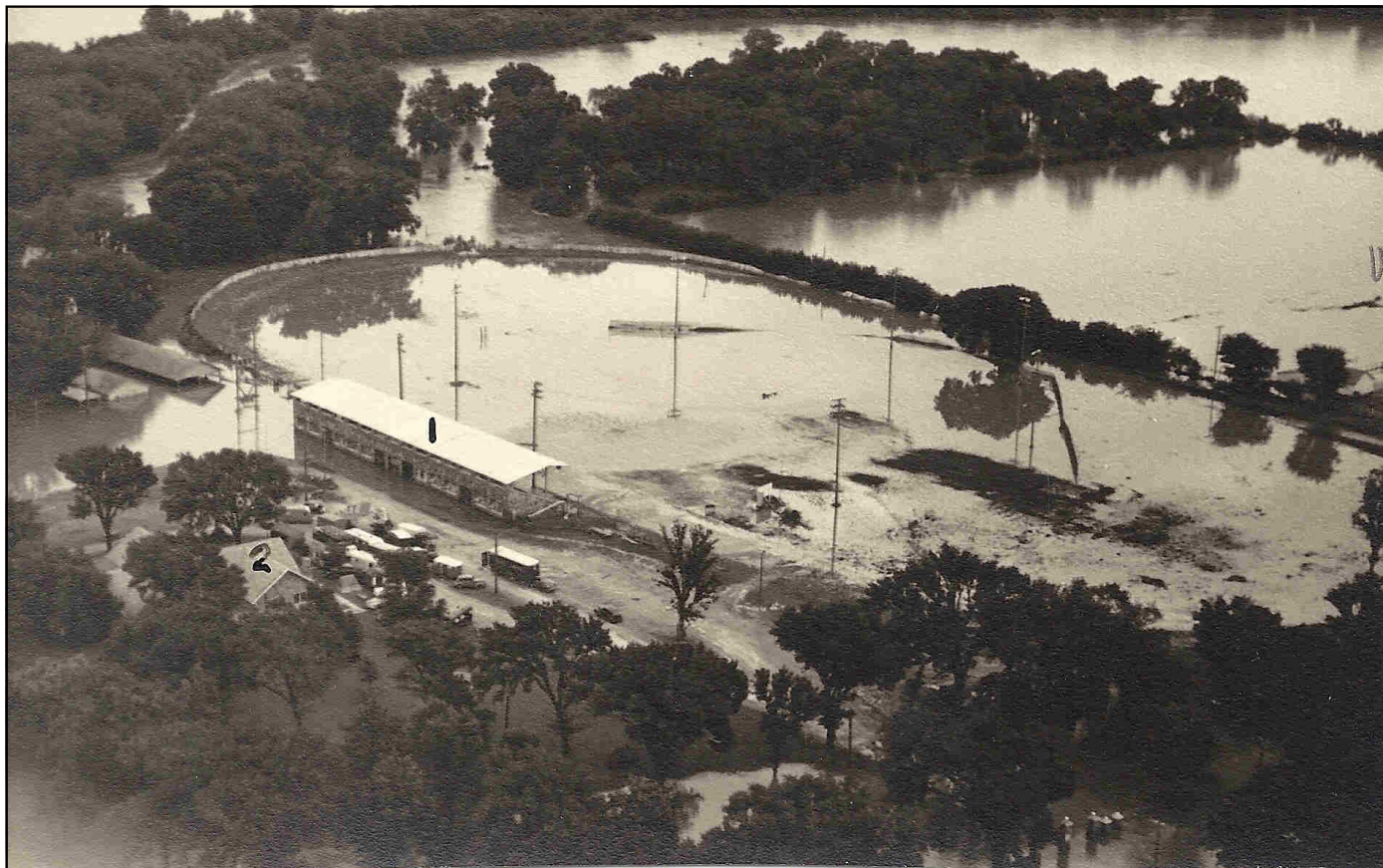
Above: Kelley Park during the 1951 flood. #1 on the picture is Memorial Stadium and #2 is the Kelley Community Hall Building. Also visible are some of the fair's livestock buildings just left of the race track. The entrance pillars for the park are in the foreground of the photograph.
