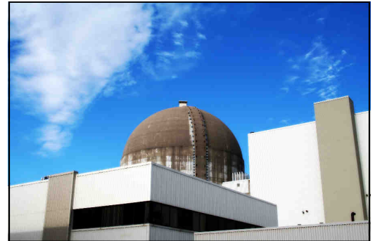
The dome is three-feet thick and the walls of the containment building are four-feet thick reinforced concrete with pre-stressed, post-tensioned rebar. The building can withstand 300 mile-per-hour winds. The building to the right of the dome is the turbine building.
