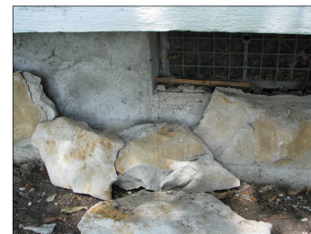
Foundation of the Church.
