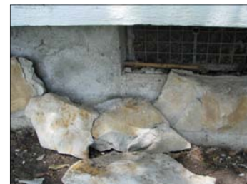
Foundation of the Church.
