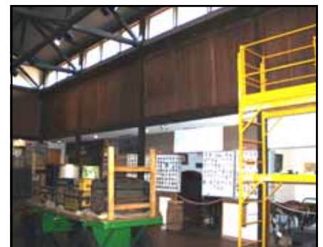
The wooden wall panels where the tools will be hung
