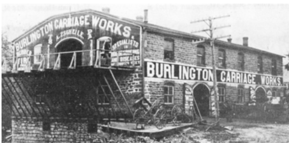
Burlington Carriage Works.
