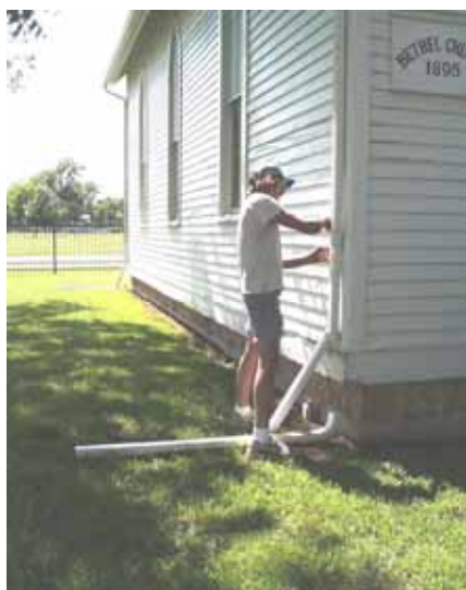
David Stratton working on the gutters.
